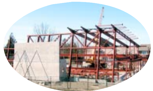
Structural of the Church 新堂結構
