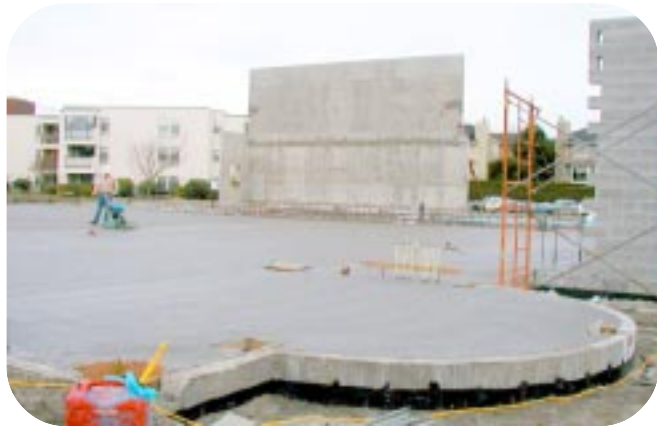
Concrete floor is almost done 混凝土地台接近完成
