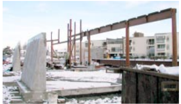
The Main Building metal frame 建築物主要鋼架
