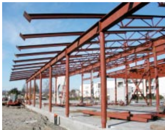
Structural steel for canopy outside classroom 課室外上蓋鋼架
