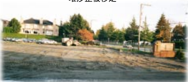
The road roller levels the ground. 壓路機縱橫，平地重現
