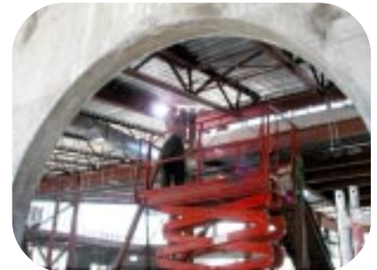
Welding Steel structure 鋼架燒焊
