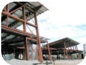
Church and Hall 聖堂禮堂外貌
