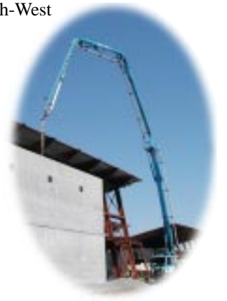
Cement work below the Sanctuary 聖所灌漿工程
