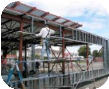
Installing metal studs for classrooms 安裝課室鐵柱
