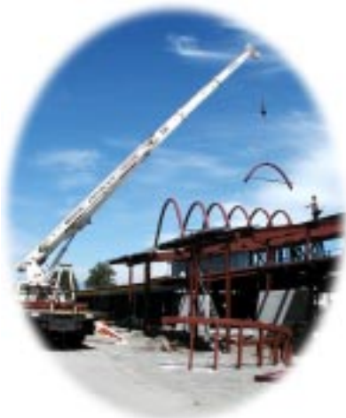
Installing arch frame for main entrance 安置正門入口拱形屋頂
